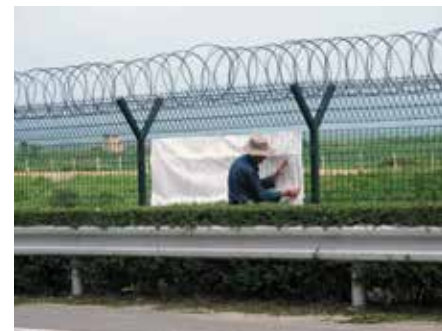
Site work at Chinese border fence, Lujiagou. Photograph: Ian Lang.
